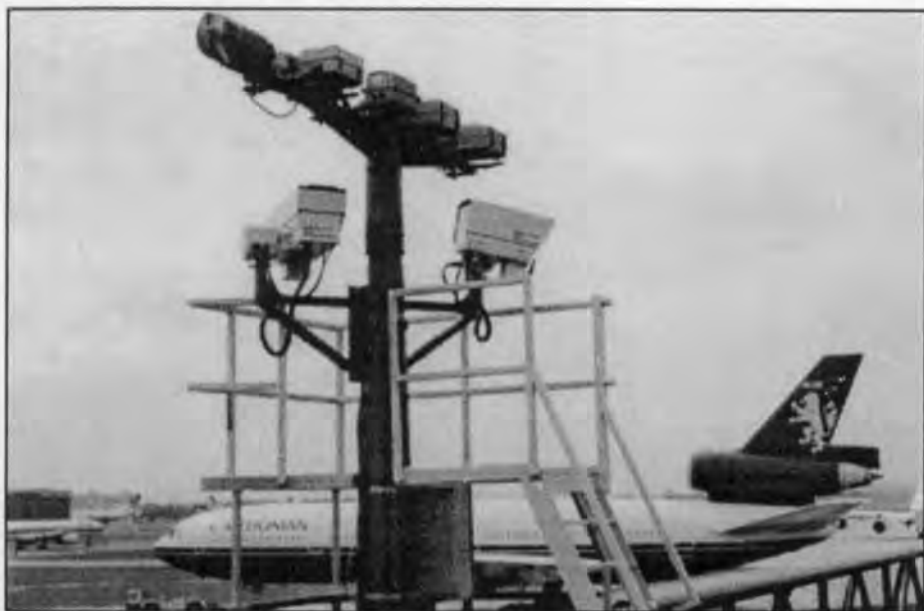
Thermovision 1000 forward looking infrared (FLIR) surveillance imager is housed in an environmental enclosure on a terminal pier several hundred feet from both the boundary edge and security control centre at London's Gatwick Airport. Second enclosure houses video camera used for daylight surveillance.
