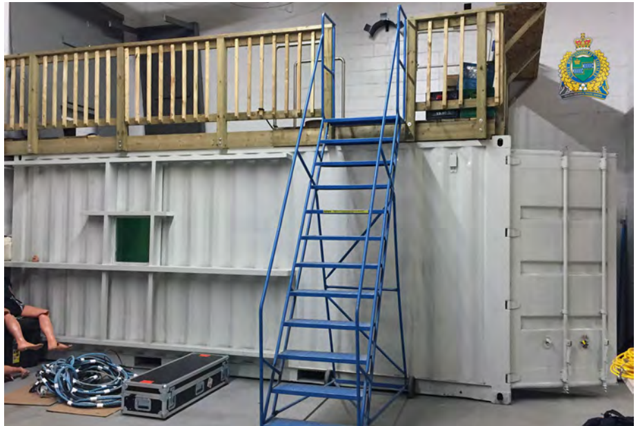
The Niagara Regional Police Service's Underwater Search and Recovery Unit has designed and built the only indoor police dive tank in Canada. The dive tank allows for the controlled training of new divers, equipment testing, hoisting and rigging, and overturned vessel entry for the rescue/recovery of trapped persons.
