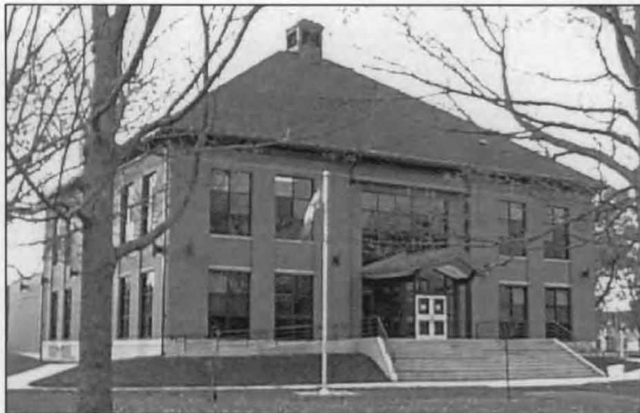
The new Truro Police building, facing the civic square park. Planned to accommodate amalgamation of adjoining communities and expected growth well into the next century, the new facility has been very well received by the community and staff.
